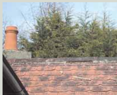
The mortar used to fix ridge tiles in place should be inspected to ensure that it has not become loose or detached
