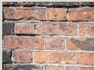
The mortar filling, or pointing, between brick or stones decays over time and needs renewal. This generally does not need to be done over an entire wall but can be confined to the areas that need it
